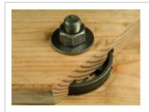
**5.** In this example, two shear plates are installed between two wooden members. The edge of one board is cut away for demonstration purposes to show the connection. Other installation options exist in which the shear plates are assembled against steel.
